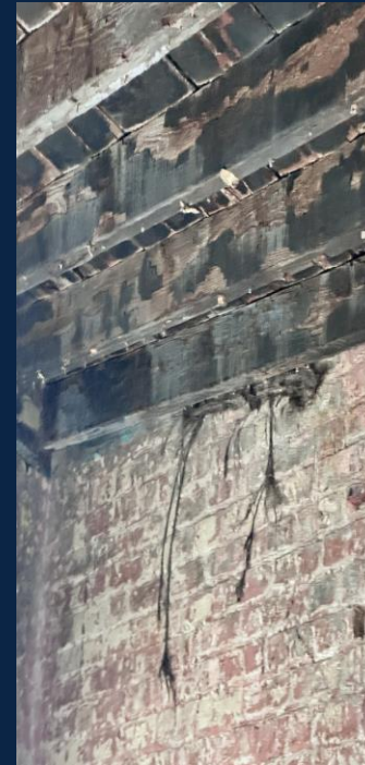
Roots growing through the second-floor wall — the condition the building had reached
